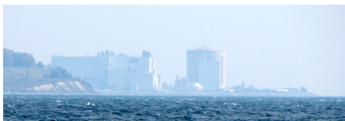
Darlington Nuclear Generating Station
