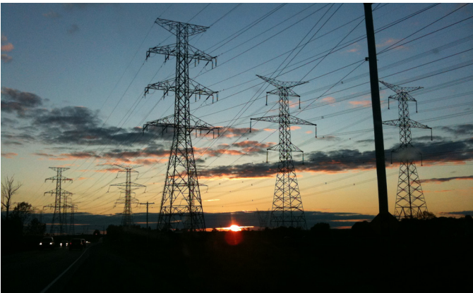
Transmission lines along Highway 7, in Brooklin, Ontario
